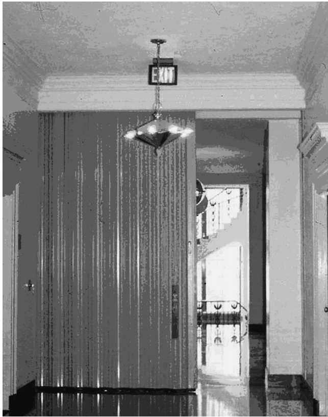
FIGURE F.2(d) Won Door in a Partially Closed Position.
