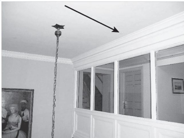
FIGURE F.3(a) Sprinklers to Maintain Glass Cooling.
