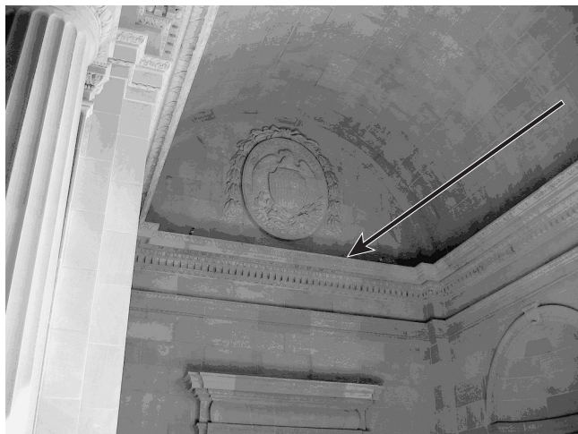
FIGURE F.3(c) Exposed Sprinkler Pipe.
