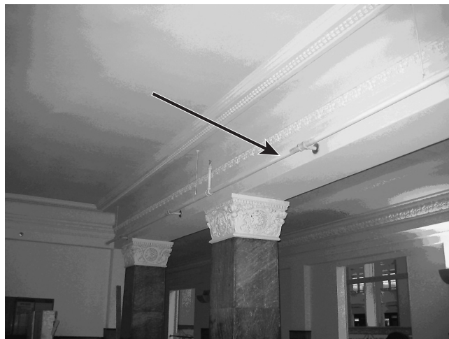
FIGURE F.3(e) Sprinkler Piping Out of Normal Sight.
