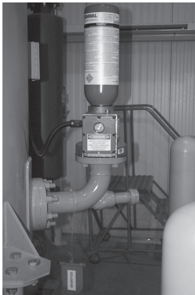
FIGURE 6.2.3.6.1.2(a) HRD Suppressor with 75 mm HRD Valve.
