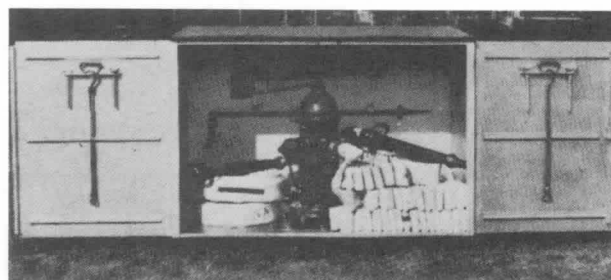
Figure A-2-3.4(a) Hose house of compact dimensions for installation over a yard hydrant. Construction may be steel or aluminum.
