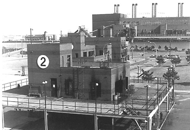
FIGURE 10.1.5 Burn Building with Raised Open-Grid Walkways Level with the Second Floor. (Courtesy of New York Fire Department Fire Academy, New York, NY.)
