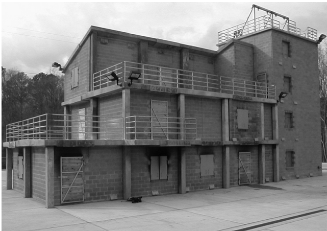
FIGURE 12.1(b) Combination Live Fire Training Structure and Drill Tower. (Courtesy of Virginia Beach Fire Training Center, Virginia Beach, VA.)
