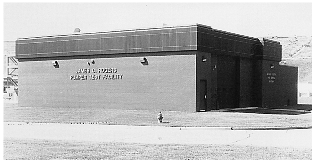
FIGURE 13.4(a) For Year-Round Testing, This Pump Testing Area Could Be Used in Cold Weather. (Courtesy of Nassau County Fire Service Academy, Old Bethpage, NY.)
