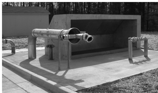
FIGURE 13.4.5 Outdoor Drafting Pit with Collection Hood. (Courtesy of Woodman Road Fire Training Center, Henrico County, VA.)
