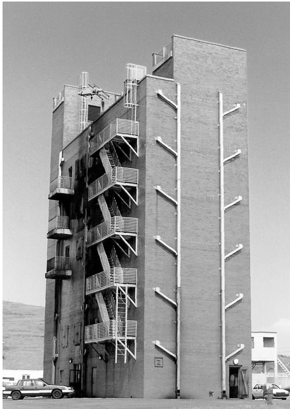
FIGURE 9.12 Drain Scuppers.
