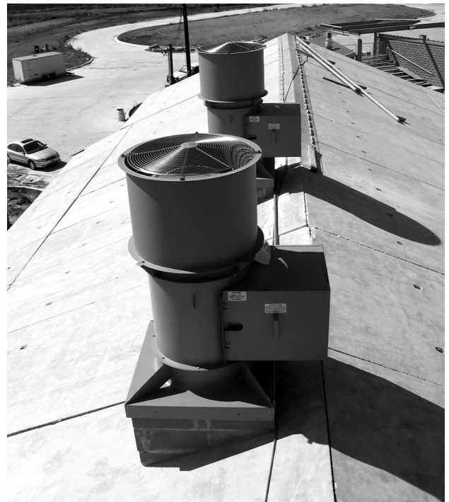
FIGURE 11.3.4 Smoke Building Exhaust Fan. (Courtesy of San Antonio Fire Department, San Antonio, TX.)
