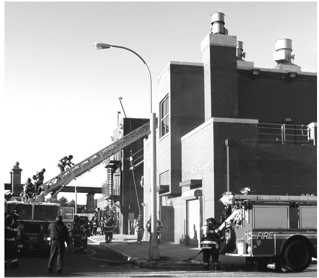
FIGURE 10.6 Gas-Fired Live Fire Training Structure. (Courtesy of FDNY.)
