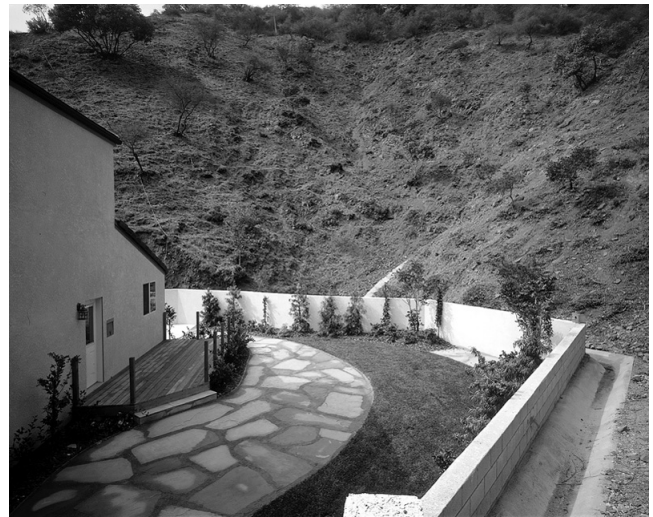
FIGURE A.5.1.3.3(b) Noncombustible Barrier Behind a House on the Edge of the Upslope. (Courtesy of Firewise Communities Program. Photo by J. Smalley.)
