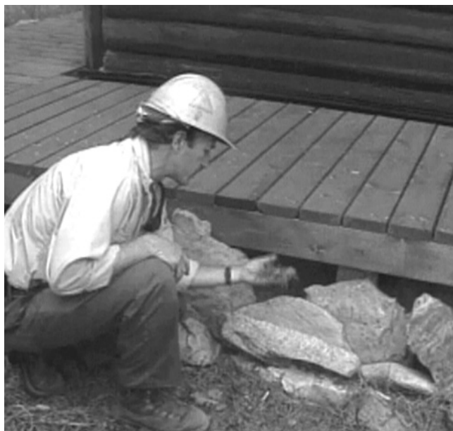
FIGURE A.4.2.4.3(a) Leaf Litter and Needles Collect in Small Spaces. (Courtesy of Firewise Communities Program.)
