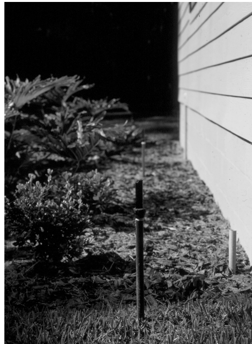
FIGURE A.4.2.4.1(b) Use of Low Volume Sprinklers in Organic Material. (Courtesy of Firewise Communities Program. Photo by G. Johnston.)
