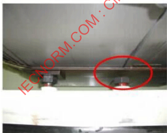
a) The foot block of bolts below iron dropped
