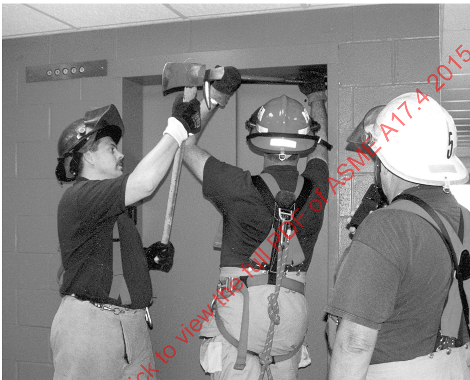
Fig. 1.3.4(f) Proper Use of Forcible Entry Tool
